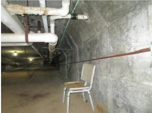
Image 17: Tunnel Corridor with Exposure To the Surge Tank
