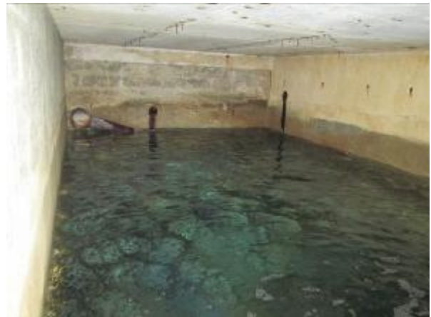
Image 93: Interior of Surge Tank
