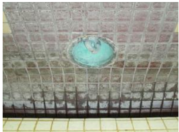
Image 31: Safety Rope Anchor
