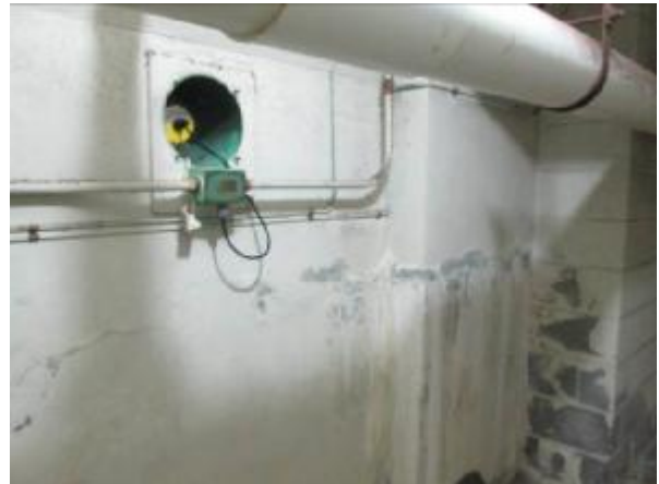
Image 10: Crack in the Pool Structure
