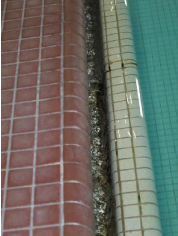
Image 23: 2" Gutter Lip Handhold
