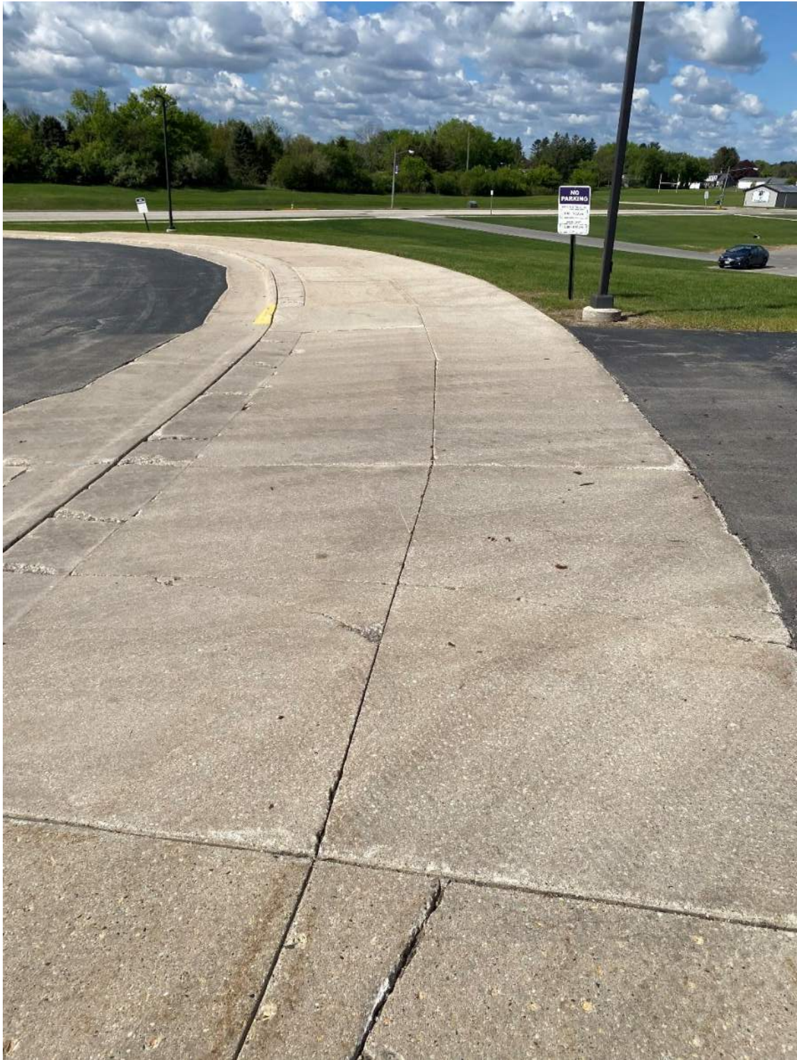
Figure 6: Cracked concrete sidewalk driveway apron into garbage dumpster area along Bus/Visitor Parking Loop.
