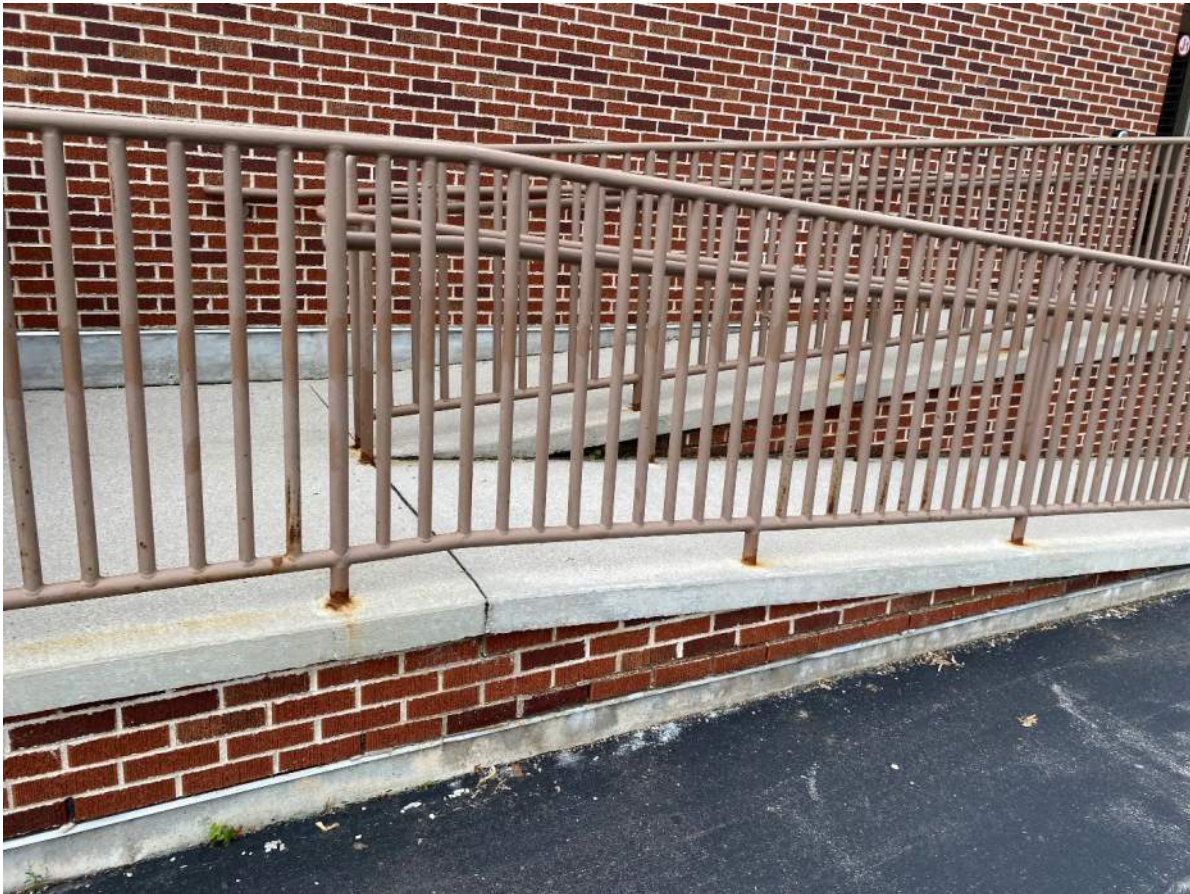
Figure 39: Back concrete ramp in fair condition.
