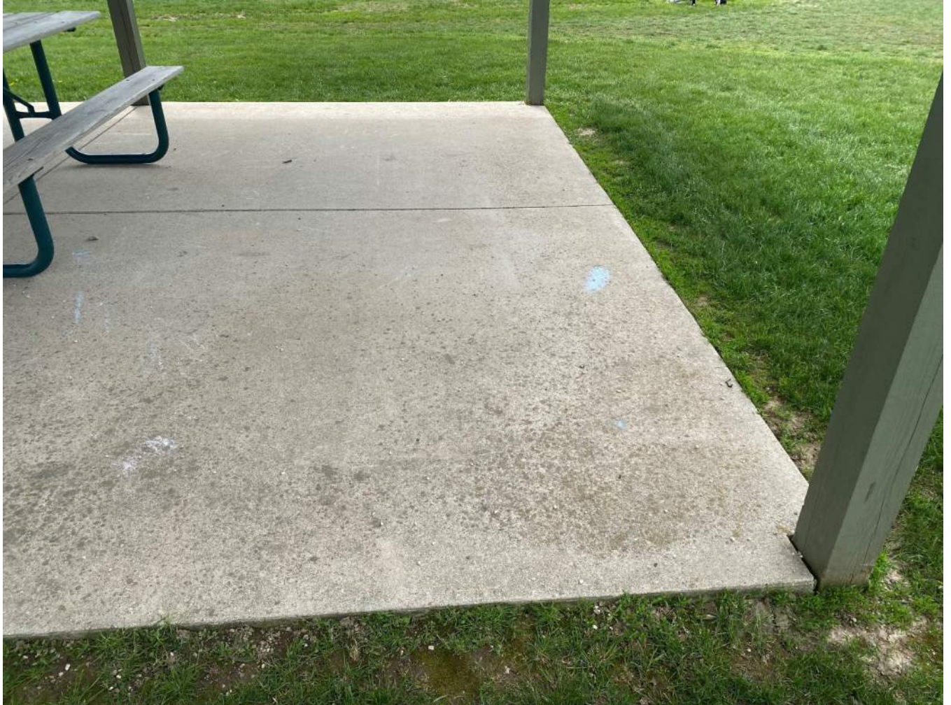
Figure 17: Concrete picnic table pad in good condition
