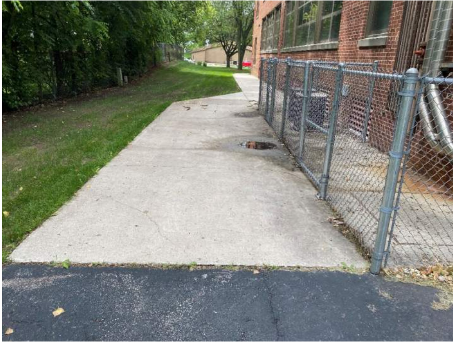
Figure 60: Cracking and settling in concrete slab on east side of school causing water to pool.
