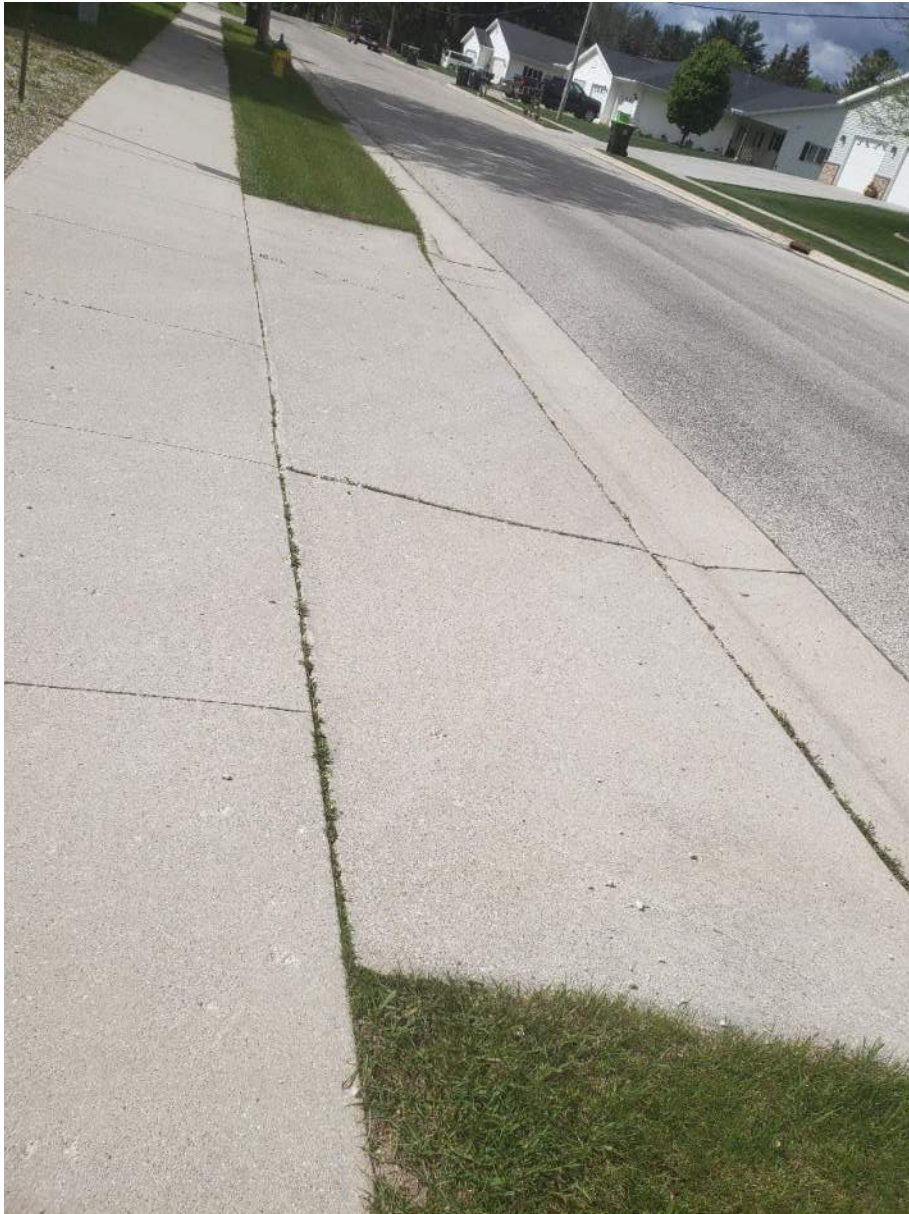
Figure 29: Driveway apron in good condition.
