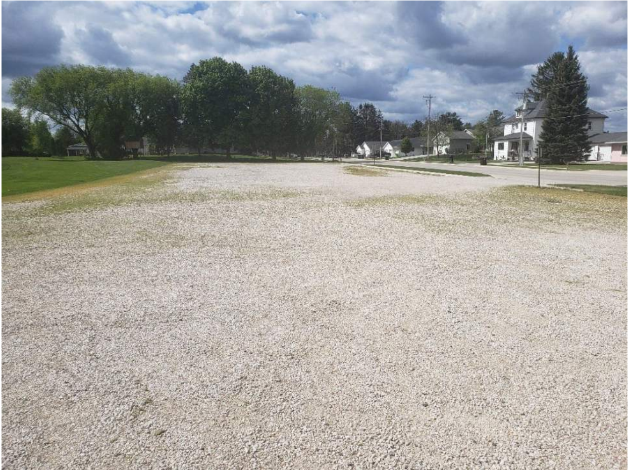
Figure 30: Gravel parking lot on South in good condition despite green growth.
