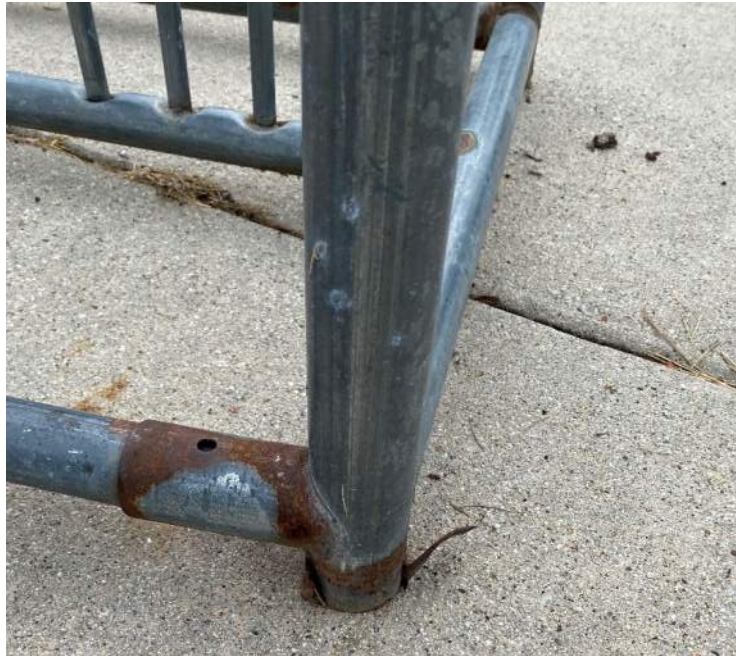
Figure 21: Sharp edges exposed on metal bike rack.
