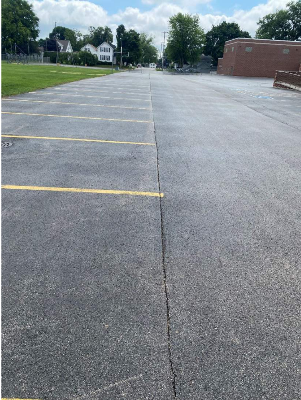
Figure 38: Newer pavement in drive lane of northwest parking lot in fair condition.
