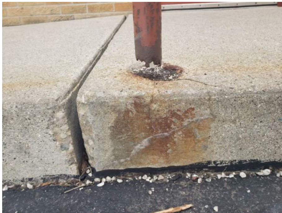
Figure 20: Severe cracking in several areas on the north ramps for existing building doors
