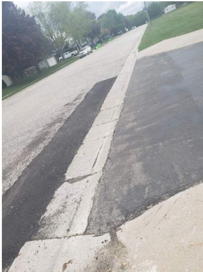
Figure 2: NW Driveway apron in fair condition.
