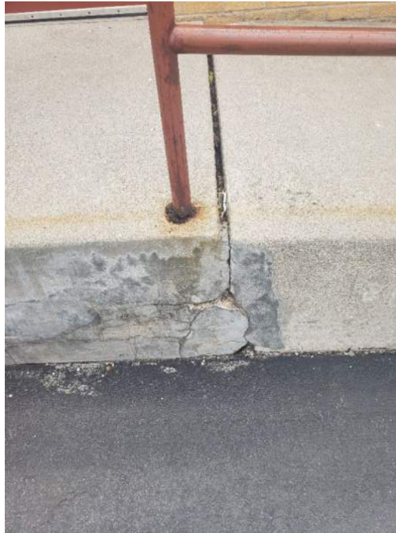
Figure 20: Severe cracking in several areas on the north ramps for existing building doors
