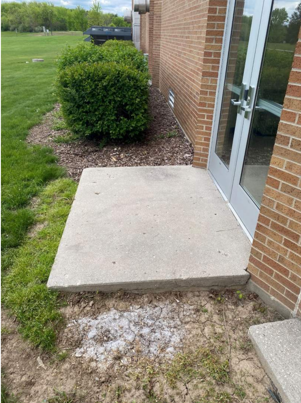
Figure 21: Door landings on east side of building
