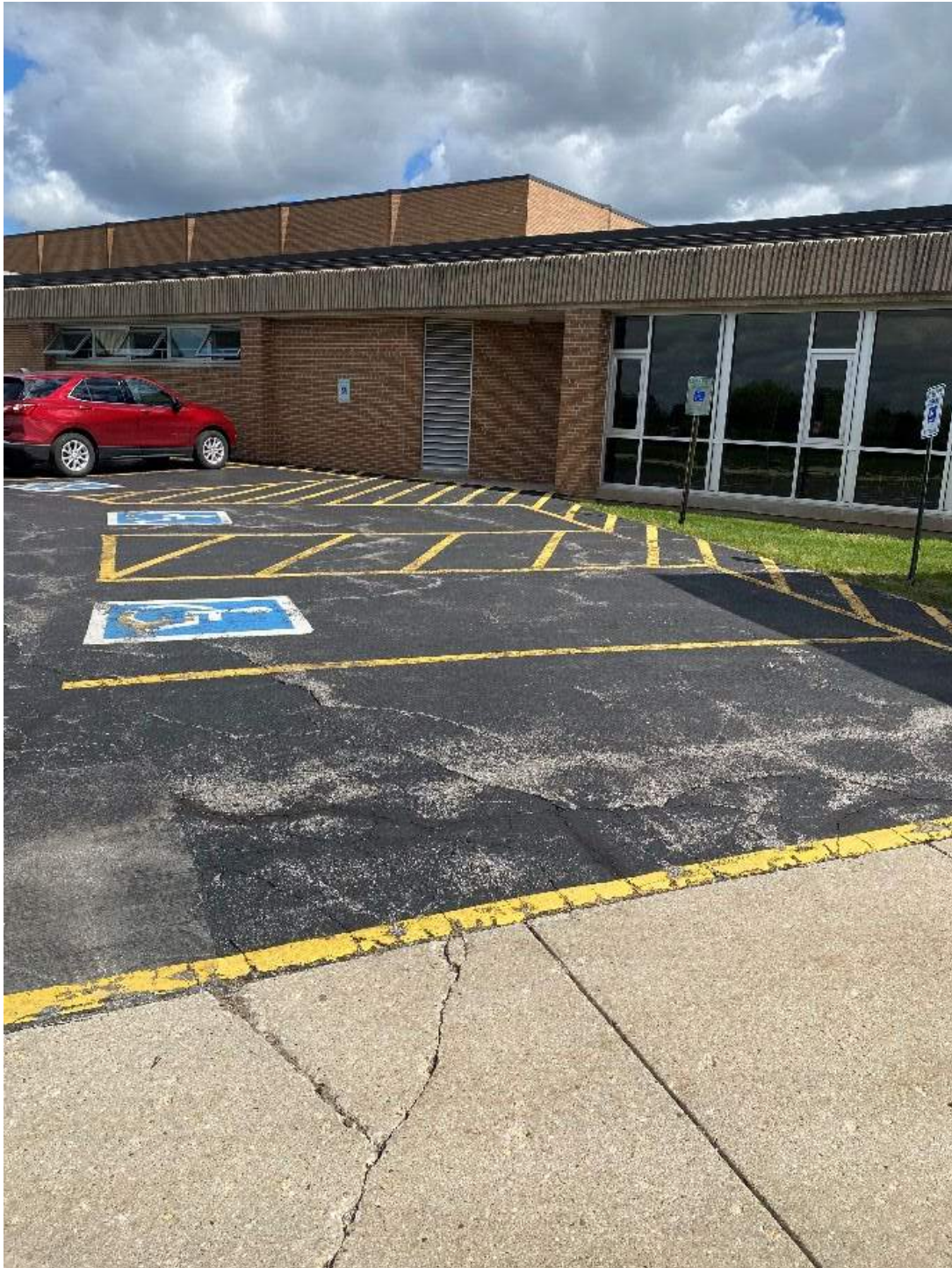
Figure 8: Pavement markings and signposts in poor condition in the Garbage Dumpster Parking Lot.
