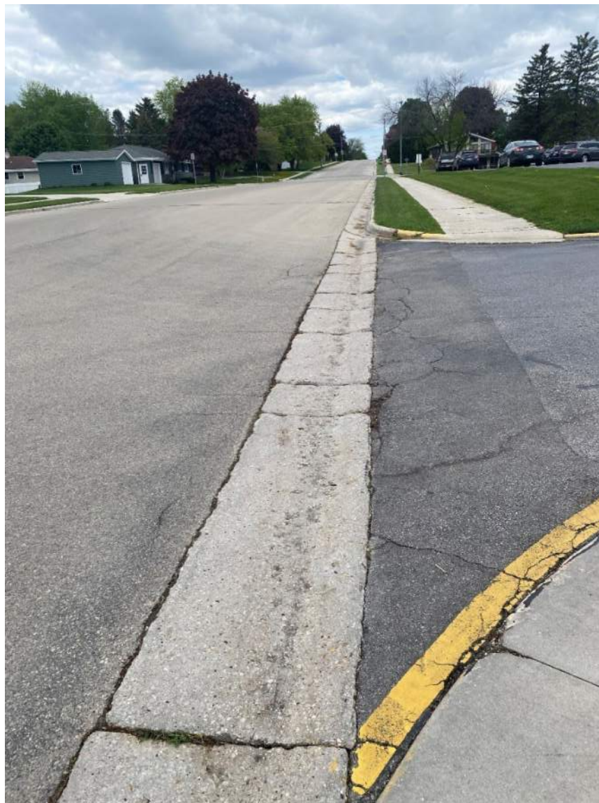
Figure 7: South driveway apron
