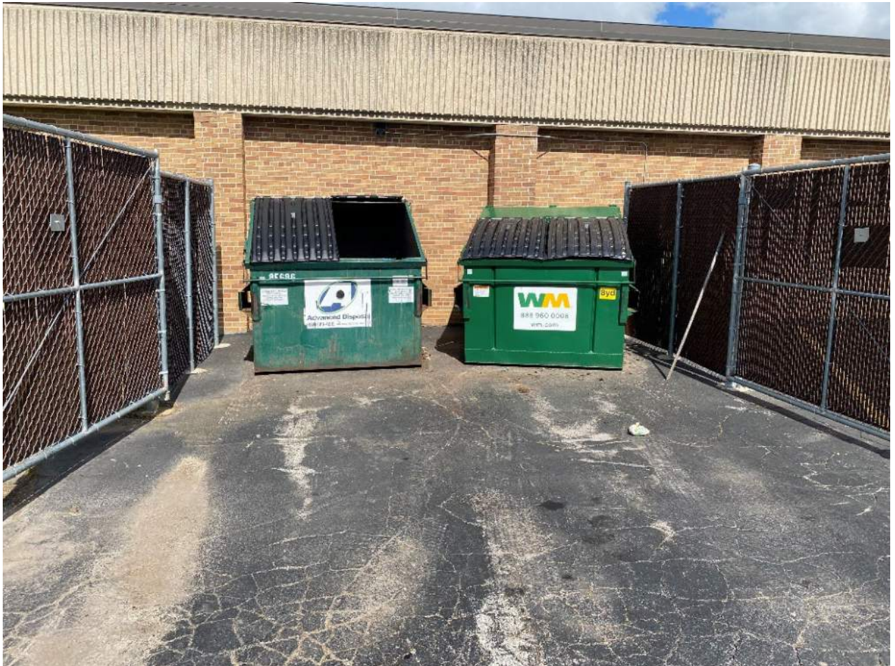
Figure 9: Dumpster enclosure fencing in good condition.
