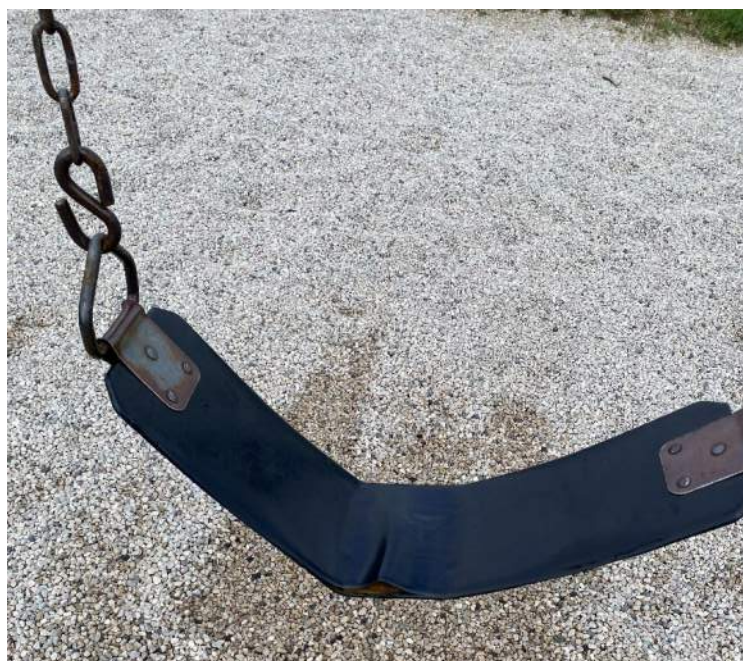
Figure 58: Broken swing seats on back swing set.
