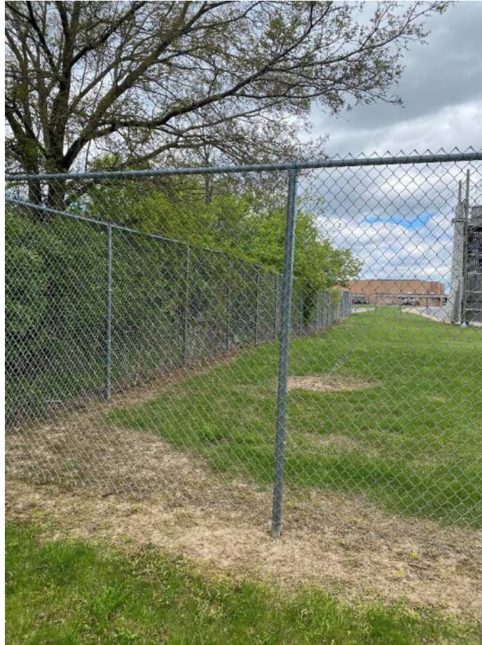
Figure 37: Trees and brush growing into fence on west side of climbing area
