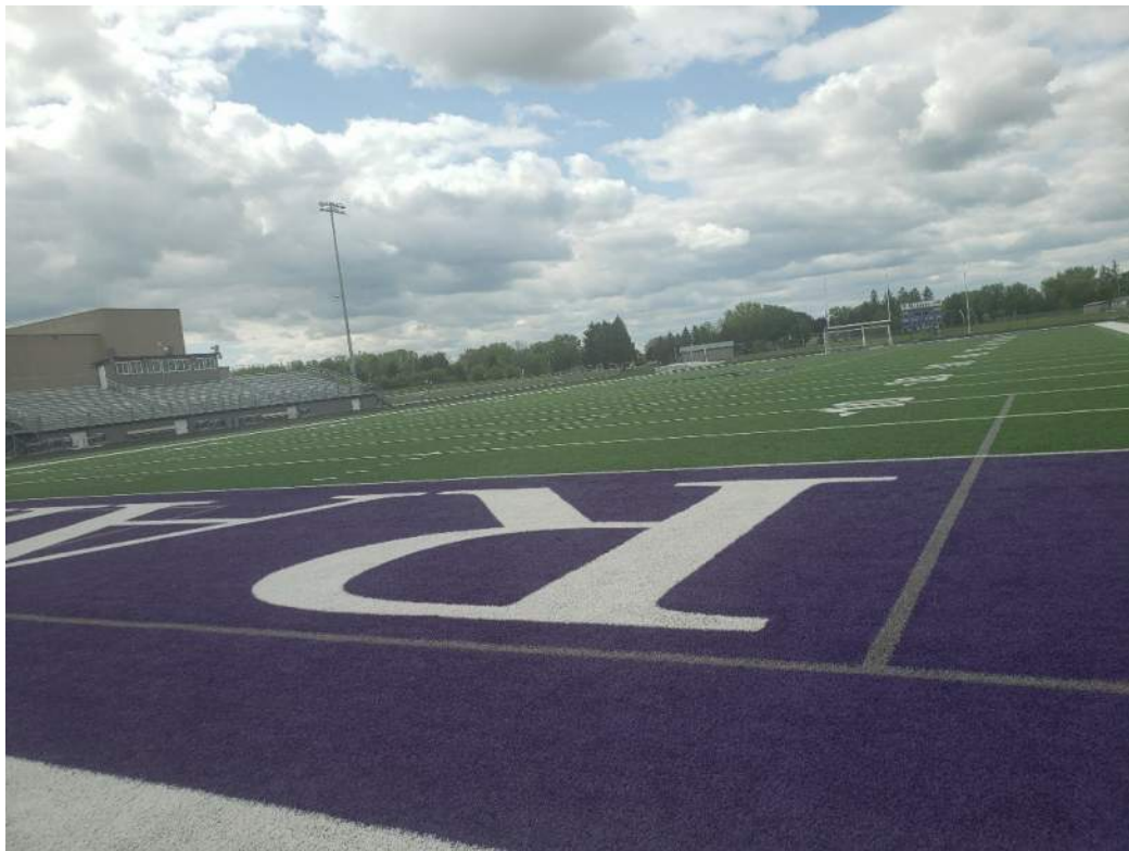
Figure 24: Artificial turf football field in excellent condition.
