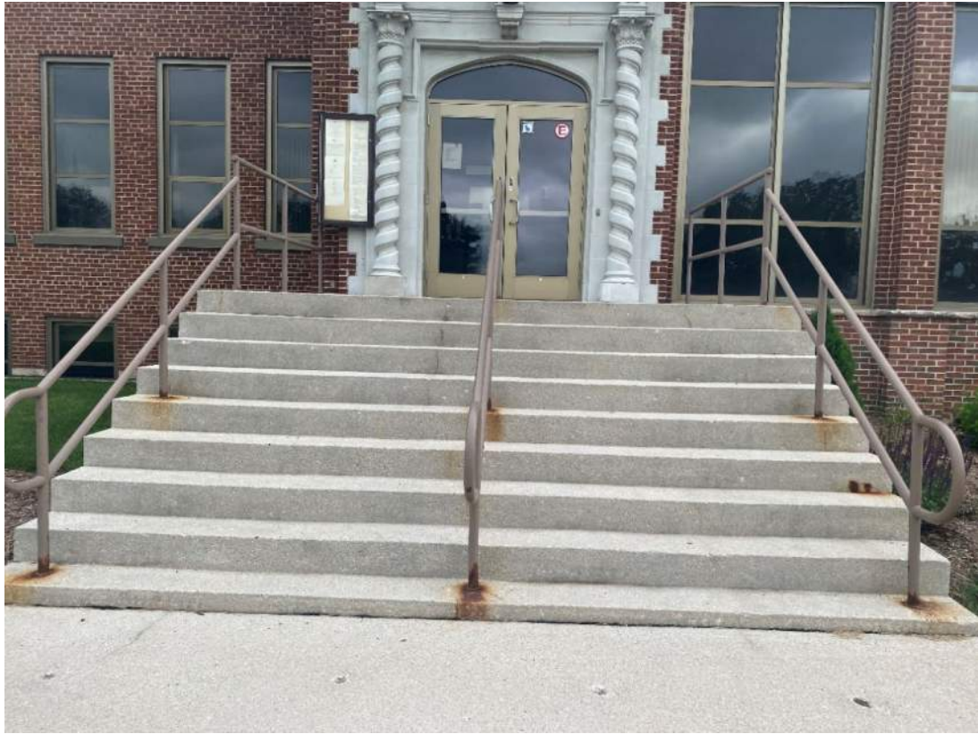
Figure 12: Front center west stairs.
