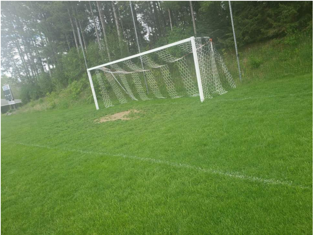
Figure 36: Dead grass in soccer field
