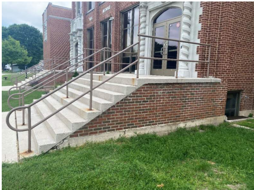
Figure 8: Side of center east concrete stairs.
