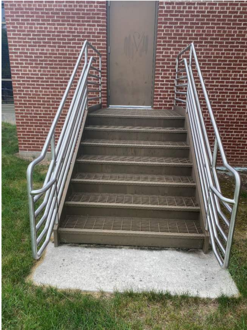
Figure 18: Front metal stair in good condition.
